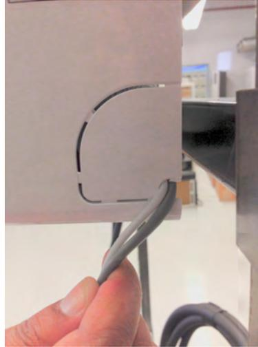
Figure 84: Indoor Unit Terminal Block with Grounding Cable (Example Only)
