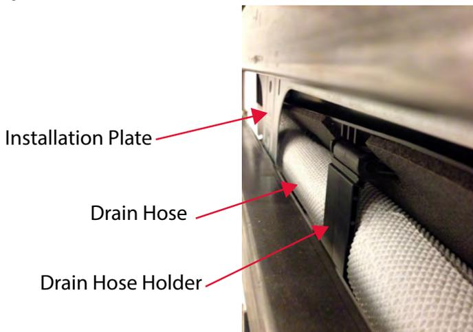
Figure 21: Mounting Unit on Installation Plate
