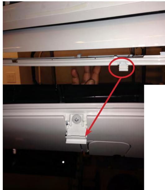
Figure 81: Remove Screws from Bottom Panel
