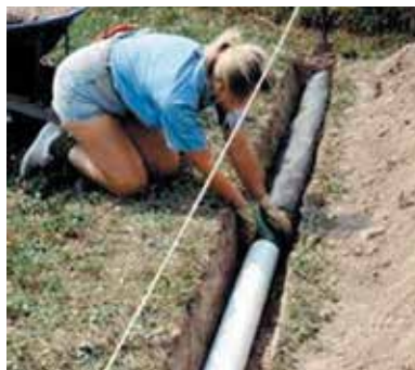
Figure 38: Underground Refrigerant Piping.
